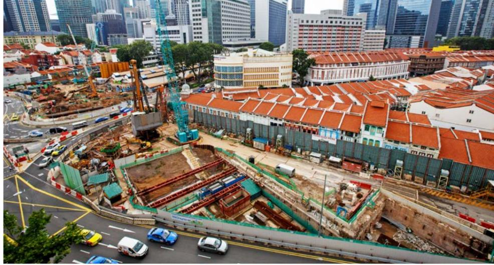
Bulk excavation and casting work carried out at the upcoming Maxwell station along the Thomson-East Coast Line.
