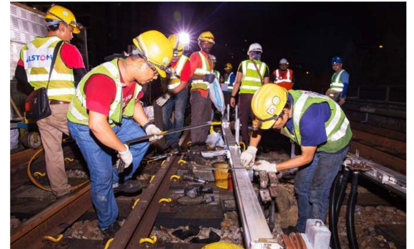
Third rail replacement works were carried out on the North-South Line for a more reliable train network. Extended engineering hours allow for renewal works to be completed faster.
