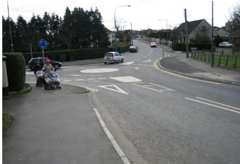
Figure 6.5 Mini-roundabout in the Lurgan, Northern Ireland
