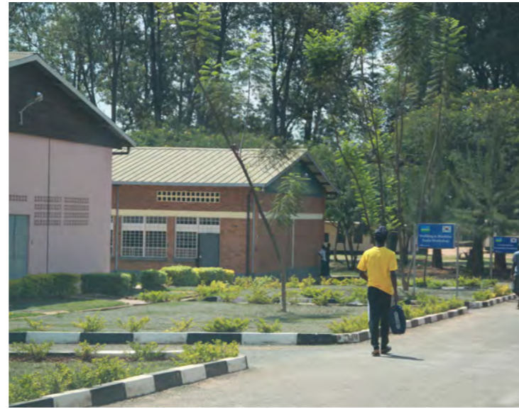
Figure 2.31 Existing Urban Road without Pedestrian Walkways
