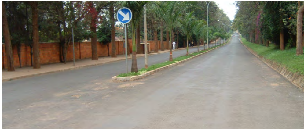
Figure 2.21 Traffic Road Markings absent from Road in Kigali
