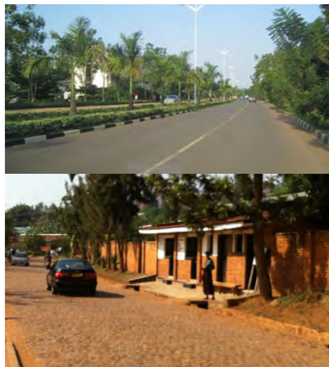
Figure 2.17 Different Pavement Types found in the City of Kigali
