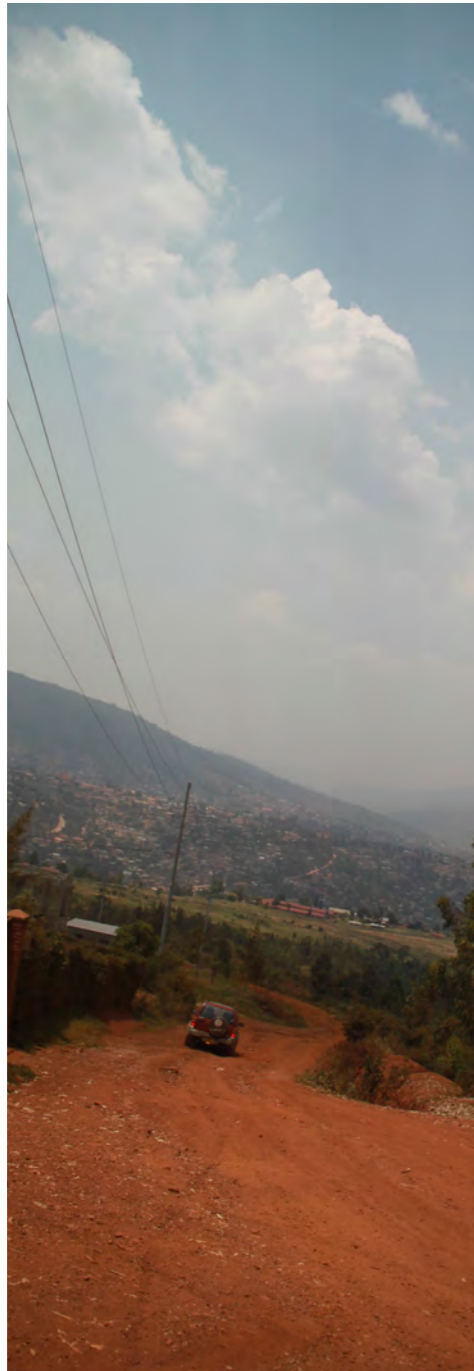
Figure 2.8 Typical Unpaved Road
