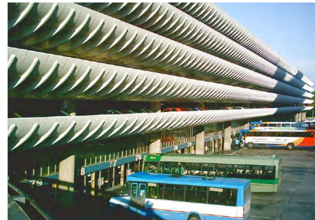
Figure 4.47 Preston Bus Station, UK, with Car Parking Facilities
