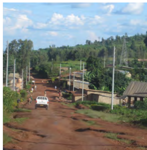
Figure 2.12 Example of Unpaved Road in Kigali
