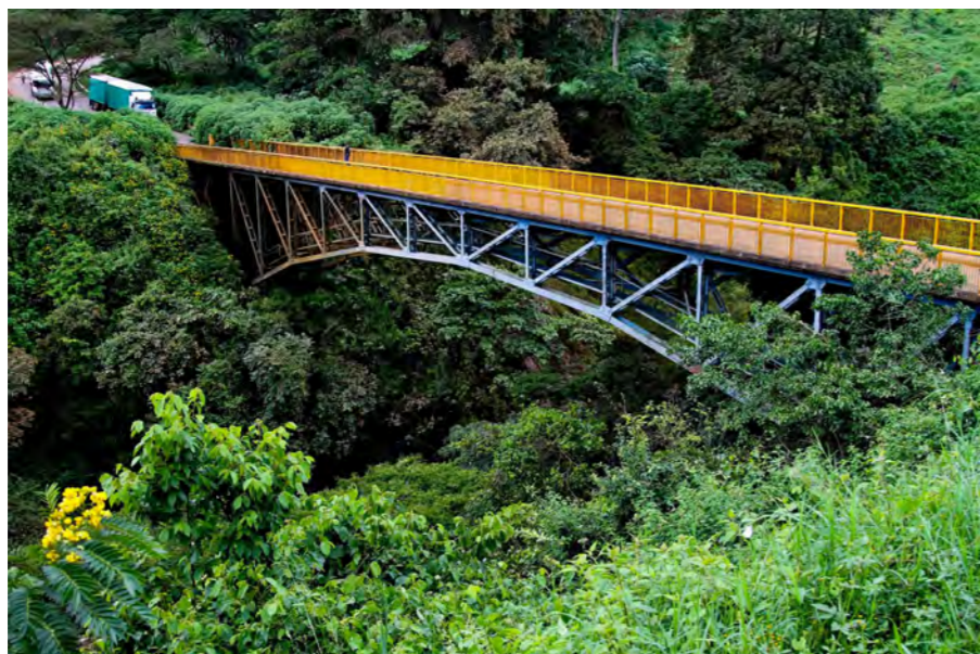
Figure 5.14 Maintenance Regime will be required for Road Structures such as Bridges
