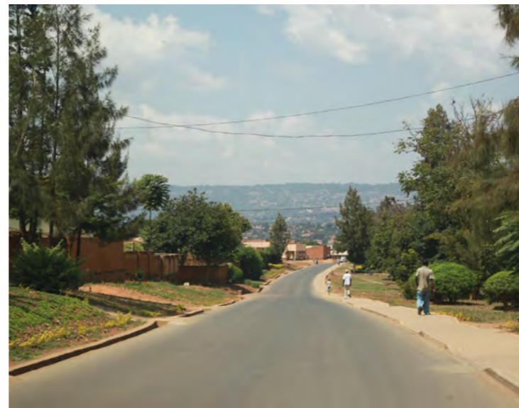
Figure 2.33 One-sided Walkway Provision
